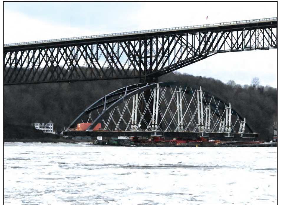
A new railway bridge section for the Portal North Bridge across the Hackensack River in New Jersey passes under Poughkeepsie’s Walkway Over the Hudson Bridge on Jan. 15 en route to its new home.
