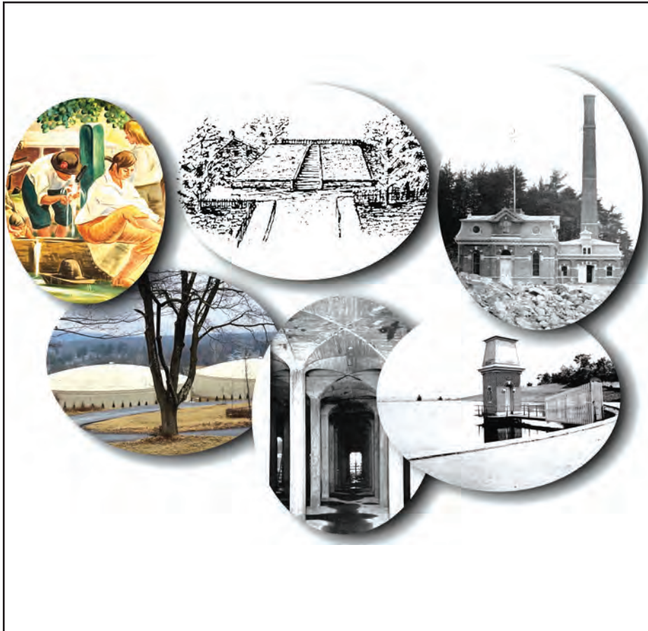
The firefighting exhibition at DCHS will feature explanations about apparatus, fire houses, and essentials like alarms and water supplies. These images clockwise from top left show: 1) image of a typical town pump that would have been used as a water source; 2) a depiction of the 1836 reservoir at Poughkeepsie's Reservoir Square, the first in the county it was designed to supported fire hydrants; 3) the pumping station that was built at the Hudson River to pump water to be stored at the top of College Hill, a practice that remains in place today; 4) the 1872 Victorian outdoor reservoir at College Hill; 5) the 1920s underground reservoir; and 6) the recently constructed water storage tanks, all on College Hill.
