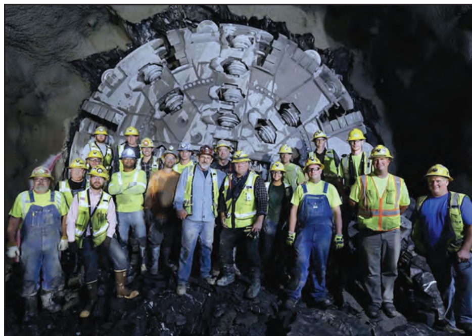
“Sandhogs” are pictured in front of the Nora underground tunnel near Chelsea, August 2019.
