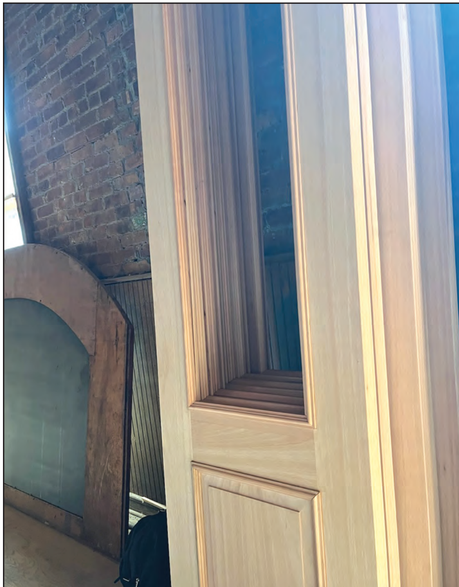
Some of the new doors that were crafted for Lyonshare Public House, which is at 246 Main St. in Beacon.
