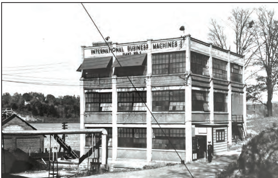
Built in 1912 for the Delapenha fruit and vegetable canning company in south Poughkeepsie, the building was bought in 1941 by a subsidiary of IBM. Initial work at the factory involved the manufacture of combat-ready light rifles or carbines. This small footprint launched IBM's massive post-war growth in the region for the next 40 years.
