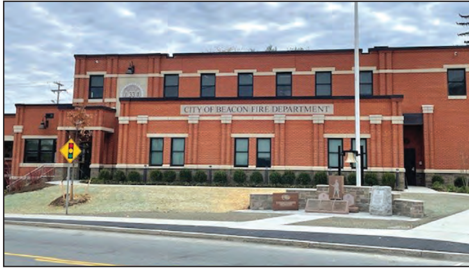
The renovated City of Beacon Firehouse on Wolcott Ave. (Route 9D), across the street from Municipal Plaza.
