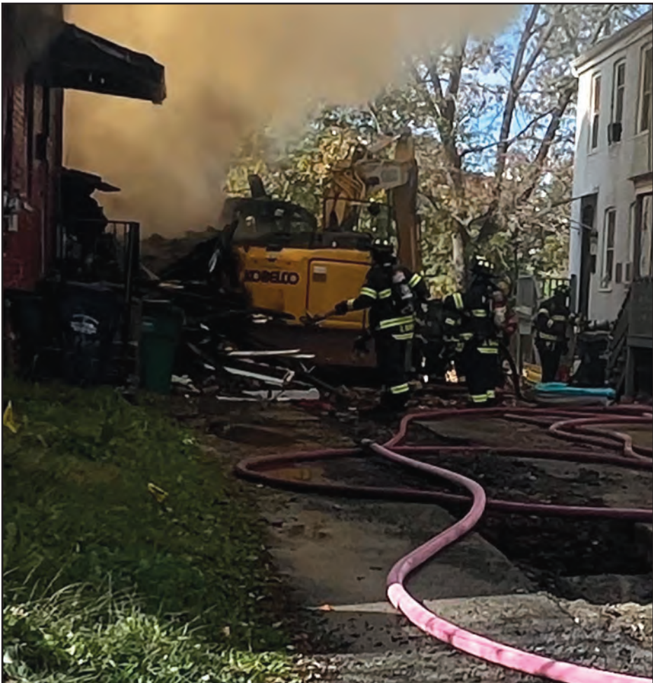
Firefighters work to put out the fire on Brick Row.
