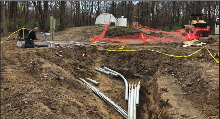
Electrical service is being installed at the Waste Water Treatment Plant in Red Hook. Courtesy photo
