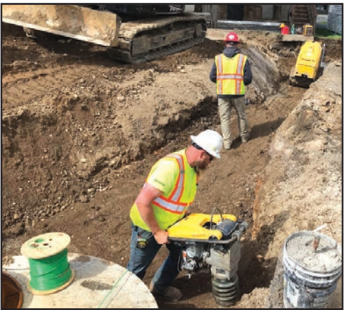
Employees work on soil compaction over a section of the forcemain of the Municipal Sewer Project in Red Hook. Courtesy photo
