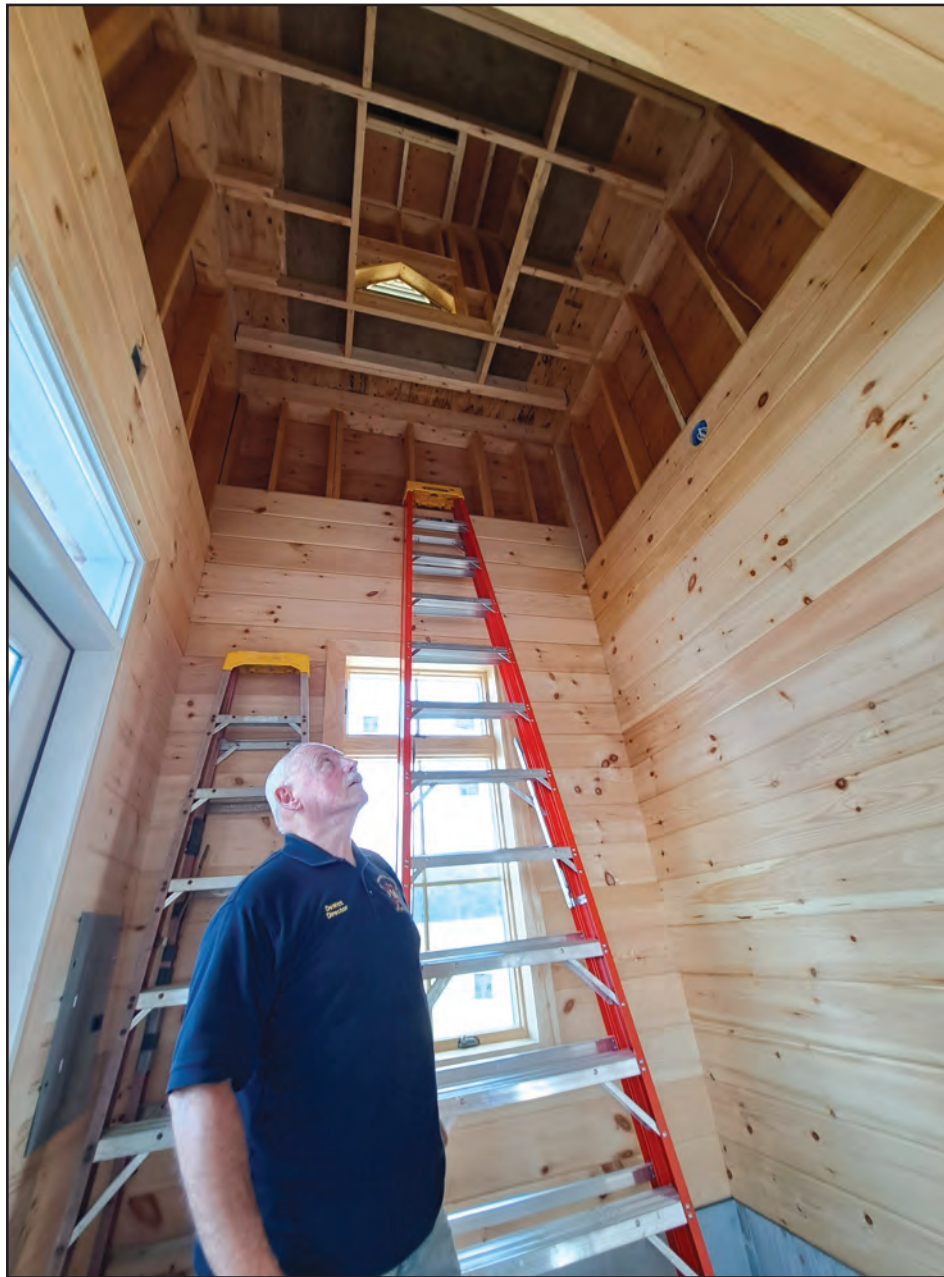
Dewitt Sagendorph of the Firefighting Museum of Dutchess County looks up into the tower of the new building at the Dutchess County Fairgrounds. The tower would have been used to hang and dry hoses after they were washed by hand around 1899-1900. Photo by Curtis Schmidt
