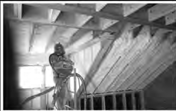
Spray Foam Insulation
