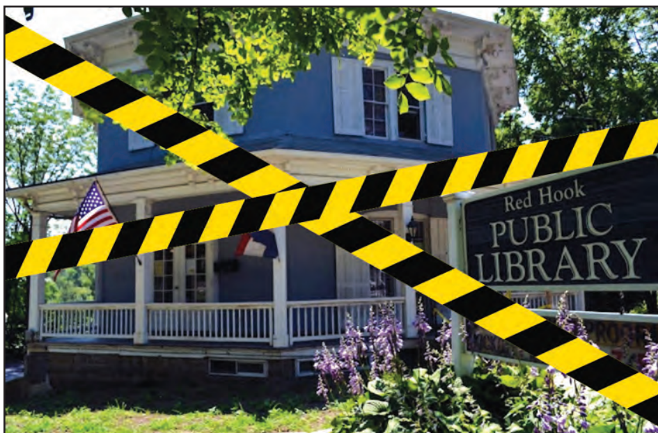
The first phase of construction at the Red Hook Library was set to begin on Sept. 23, starting with the front porch. Courtesy photo
