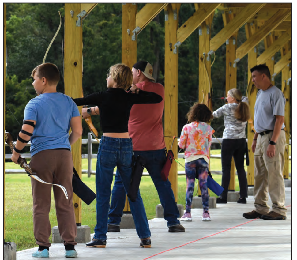
The new archery range at Bowdoin Park doubles participant capacity with space for 20 people to take part per session. The range features a covered firing line and storage shed for equipment. It is located adjacent to Pavilion 4 and features an accessible sidewalk and parking area, making the program easy to access for participants of all abilities. Courtesy photo
