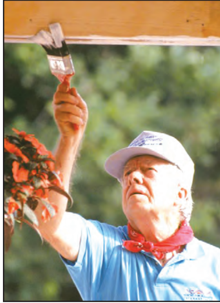
President Jimmy Carter paints one of the many Habitat for Humanity houses he helped to build.
