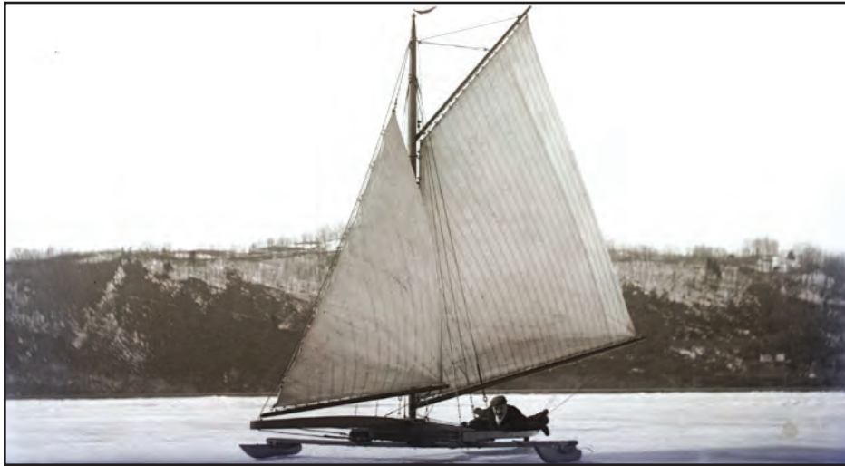
In this 1901 photo on the Hudson River, the unnamed operator lies flat on the ice yacht to minimize any air resistance that sitting up would create. Able to reach speeds of 100 miles per hour, these "boats or yachts" were for a time, the fastest (if very limited) means of travel.
