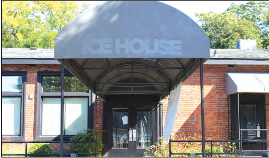
The former Ice House in the City of Poughkeepsie.
