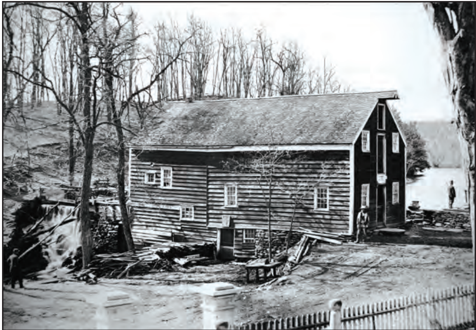
The Ward family of Pleasant Valley had active orchards and livestock, and operated this mill which was directly opposite their home.
