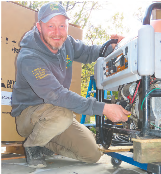
DS Home Services provides maintenance for all generators. Above is technician Thomas Lievers. Below: DS Home Services provides Fall checks on all HVAC units. Photo by Curtis Schmidt and courtesy photo
